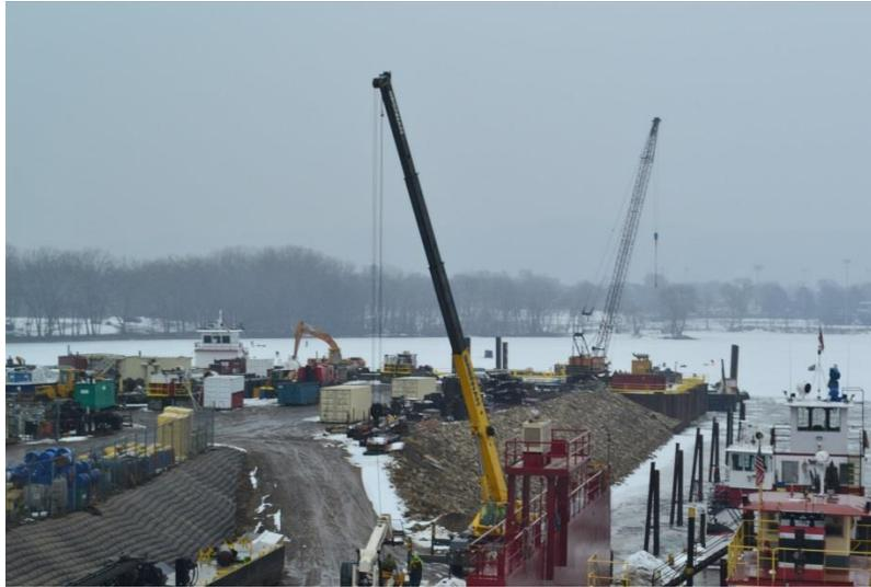
Figure 8 J.F. Brennan Company's south shore and open storage. Rock riprap and dolphins.
